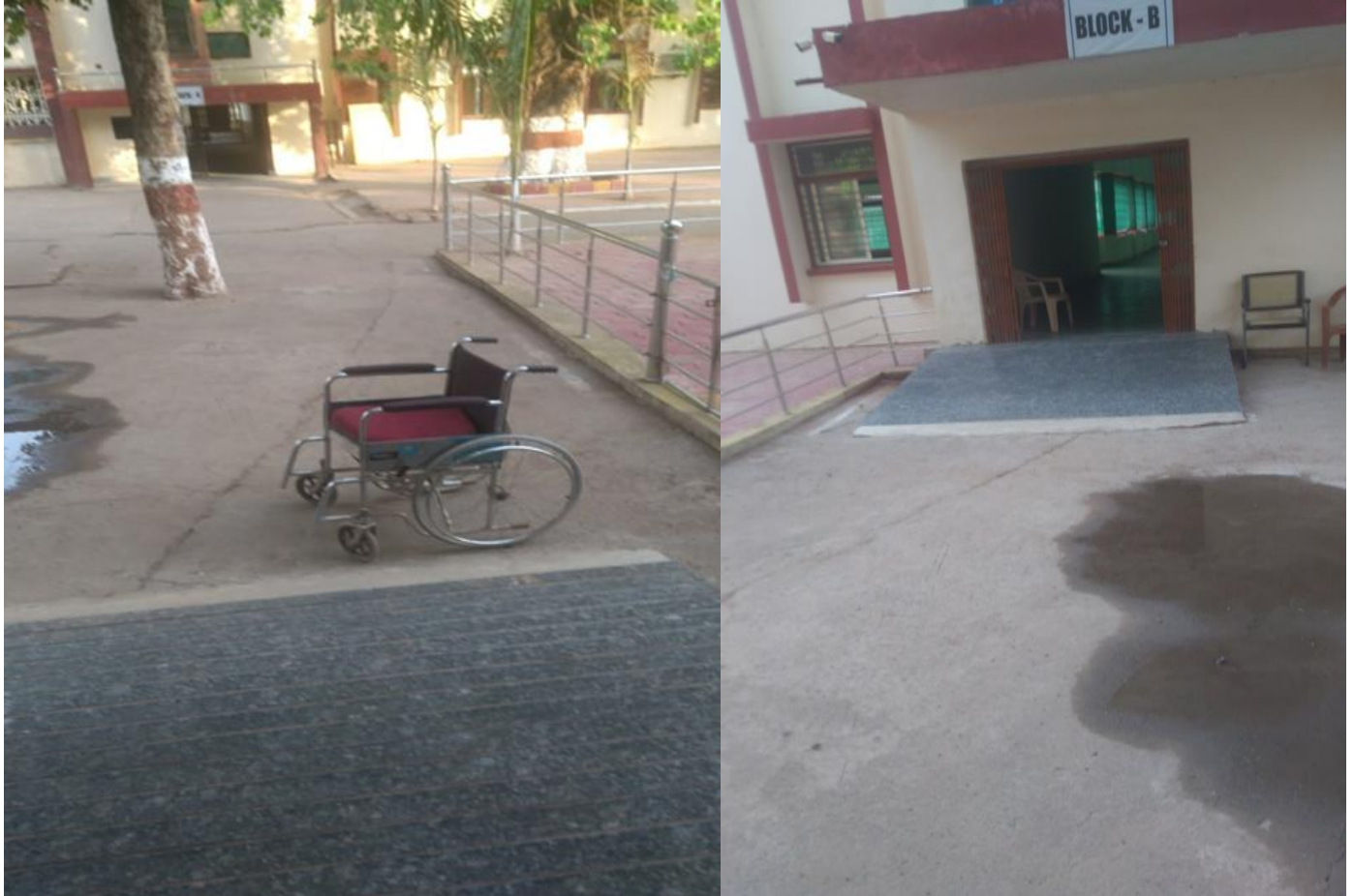
Pic 12 Wheel Chair & Ramp Facility for disabled students
