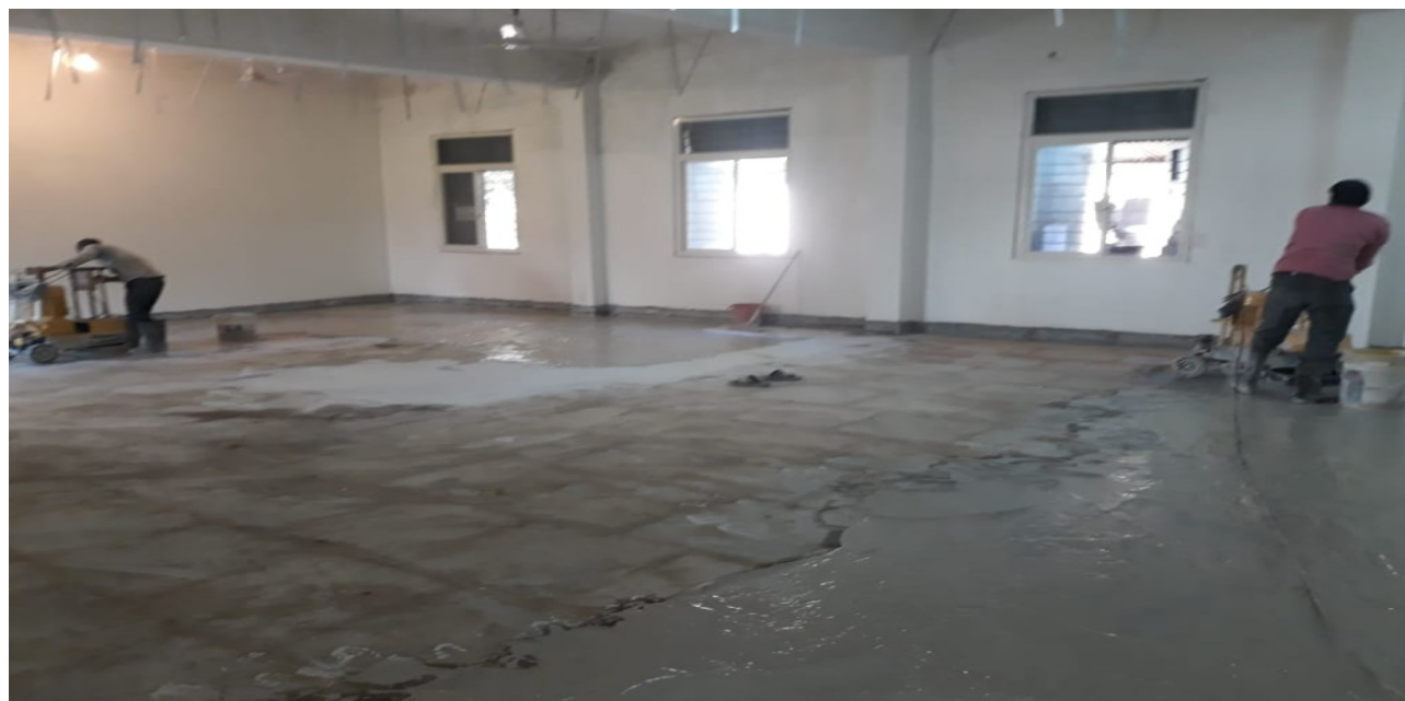
Pic Class Room Construction Regarding World Bank
