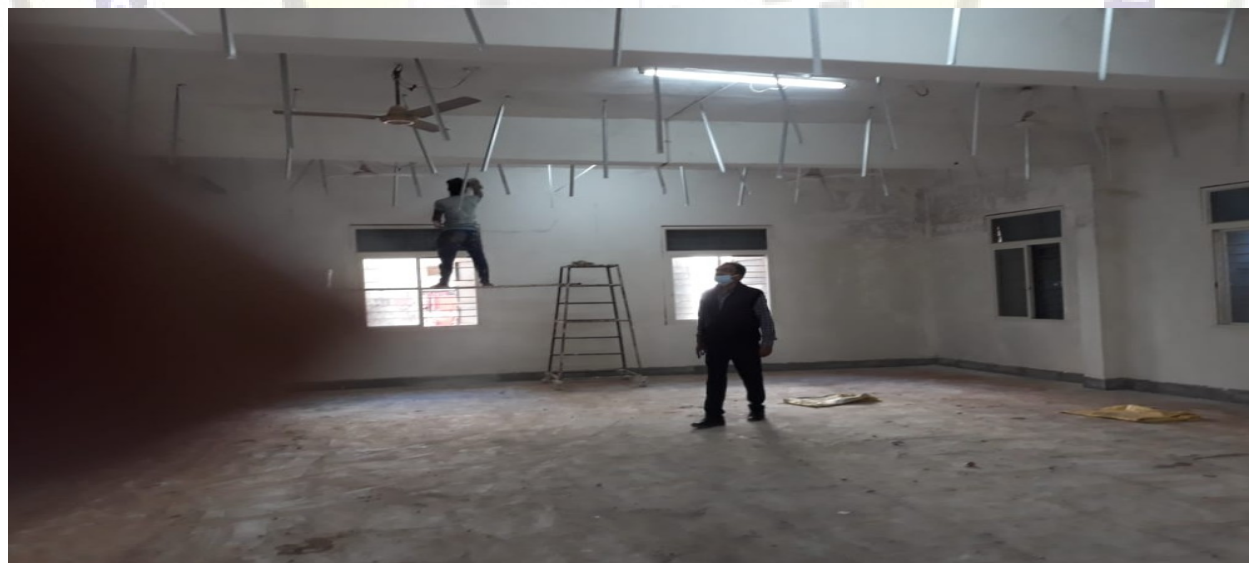
Pic Class Room Construction Regarding World Bank
